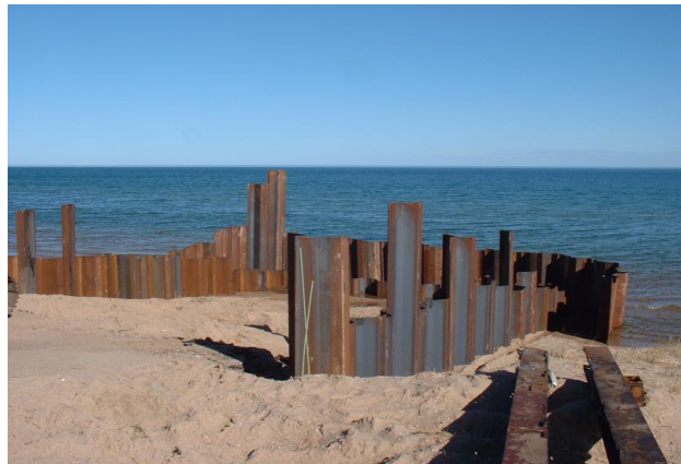
This cofferdam was used early in the construction to keep the concrete wave-free while it sets.
